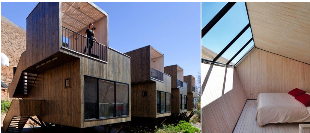
Figure 10: Hotel Elqui Domos – Cabin lodges
